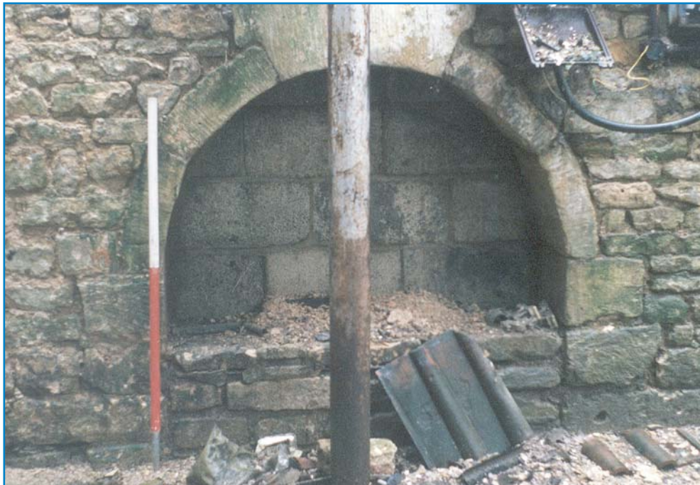
Plate 5: Building 2b, detail of furnace
