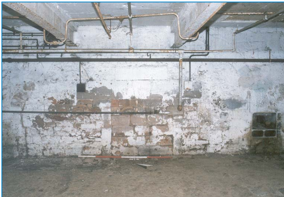
Plate 13: Building 5b, west elevation detail showing blocked opening and wheel mountings in east wall of overshoot building
