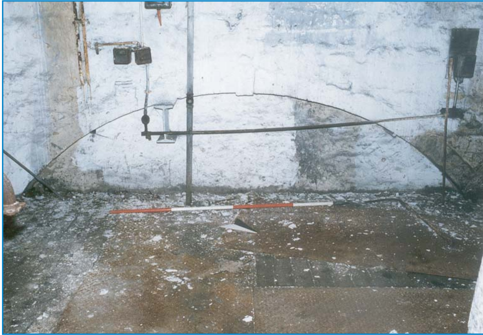
Plate 14: Building 5b, detail of upper part of wheel housing (internal face of west wall)
