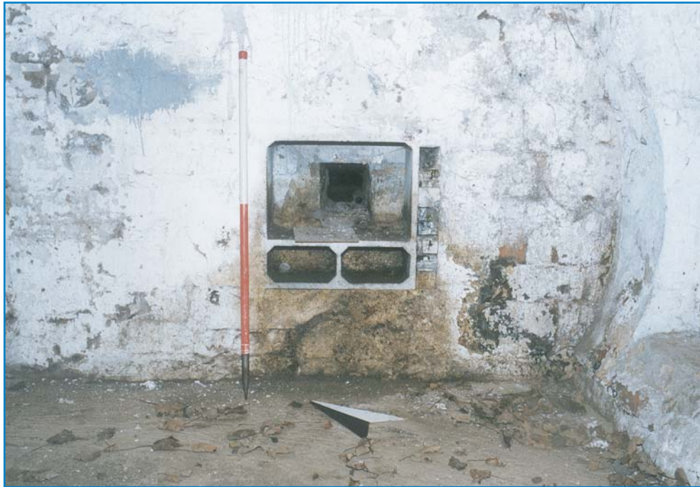
Plate 12: Building 5b, detail of wheel mountings and housing in east wall of overshoot building
